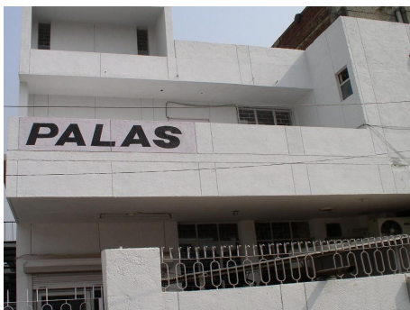
Easily Accessible Location
